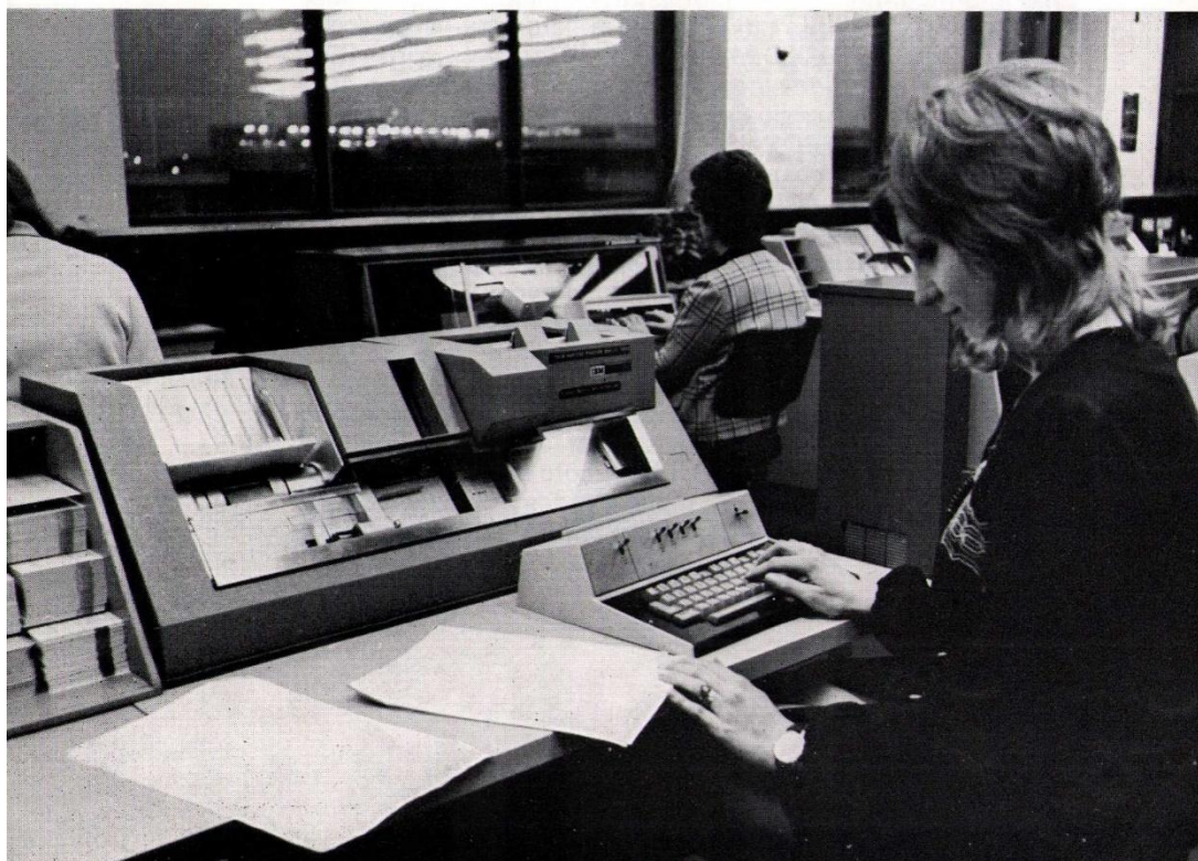
Card punch in Data Preparation Room
