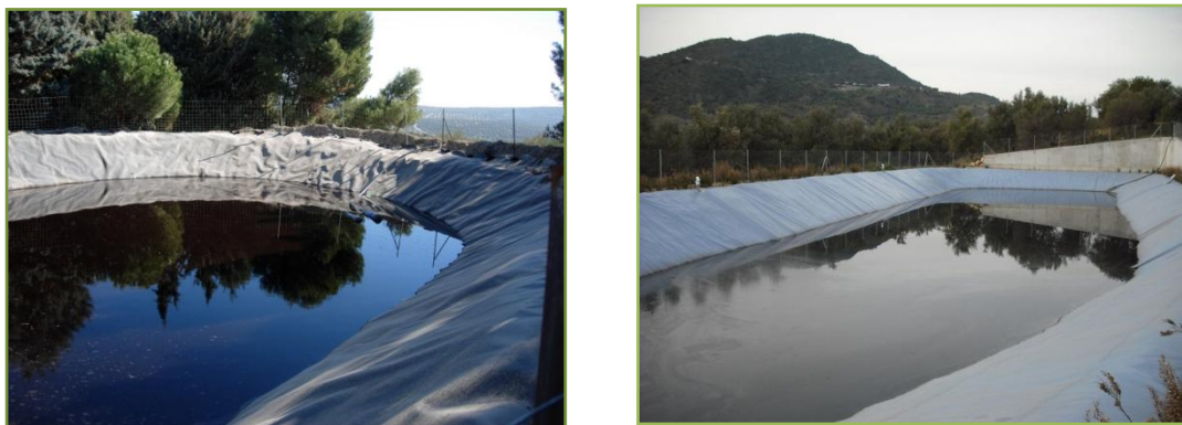
Fig. 1. Ponds for storage and natural evaporation of olive mill effluents.
