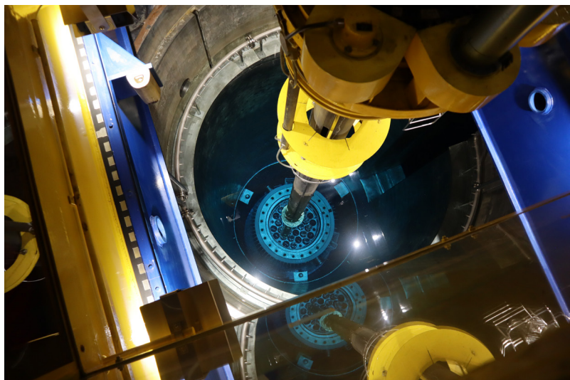
Loading of the first Westinghouse NOVA E-6 assemblies into Loviisa-2 core in August 2024
