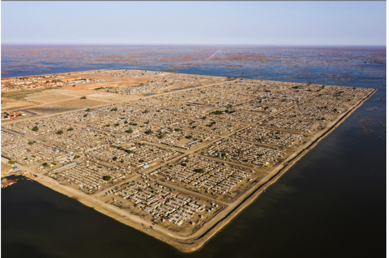
Photo: Dykes protect the main IDP (internally displaced persons) camp in Bentiu.© UNHCR/Andrew McConnell
