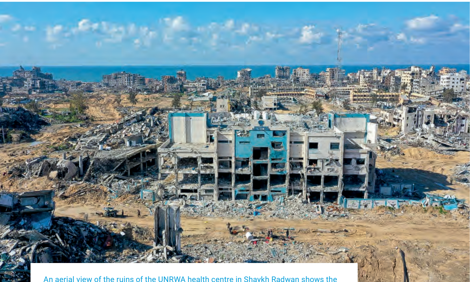
An aerial view of the ruins of the UNRWA health centre in Shaykh Radwan shows the extent of widespread destruction in the Gaza Strip since October 2023.
